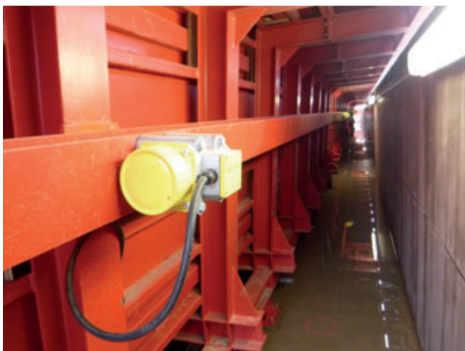
The formwork before the modifications
