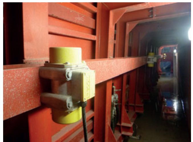
The formwork after the modifications
