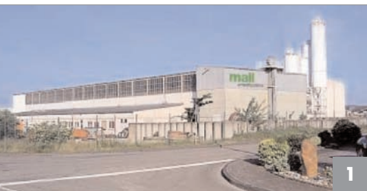
The company Mall Umweltsysteme GmbH in Nottuln, Germany
