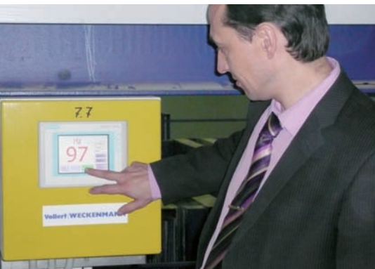
Fig. 8: Project manager Alexander D. Jaroshenko (DSK Blok) operates the vibration compaction via one of the new Brecon touch panels.
