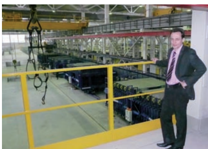
Fig. 10: The project manager Alexander D. Jaroshenko from DSK Blok is pleased with the clean, tidy installation
