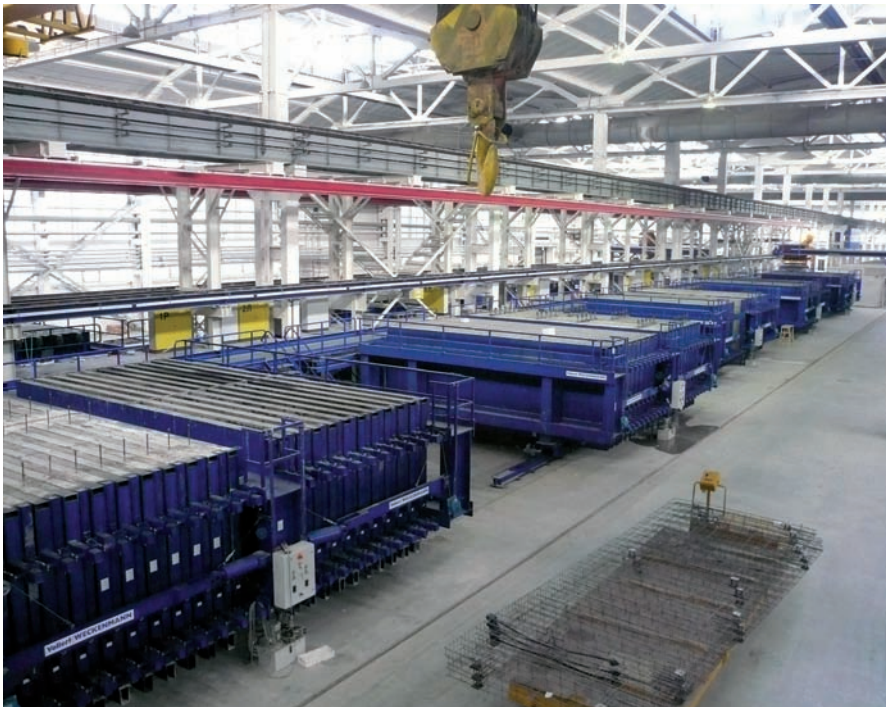
Fig. 1: The control equipment for the vibration of five battery formworks with almost 500 vibrators is installed on a railing at a height of 4 metres. All five control units can mutually replace each other without switching over (redundancy).
